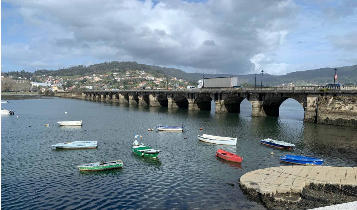
A medieval bridge on the Camino in Spain.
